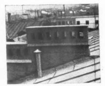
Fig. 7, a group of roof terminals to internal bathrooms of a block of flats.
