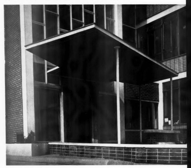
The canopy, supported outside by three slender steel columns, is also supported behind the glazing.
