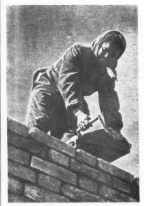
Fig. 4, bricklaying in the USSR; the first member of the bricklaying team pouring mortar on to the wall.
