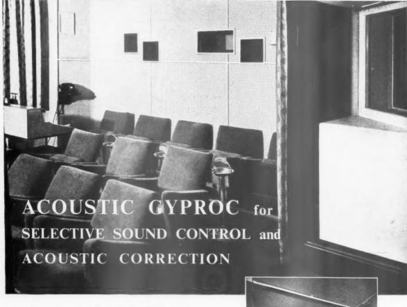
For walls and ceilings at the B.B.C. Studios, Maida Vale, Acoustic Gyproc with a 1" bitumen bonded Fibreglass backing has been used. Above, a section of the Private Theatre and, right, the ceiling in the Projection Room.
