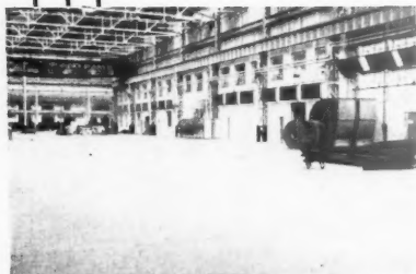
GRANOLITHIC FLOORING IN AN ALUMINIUM WORKS
