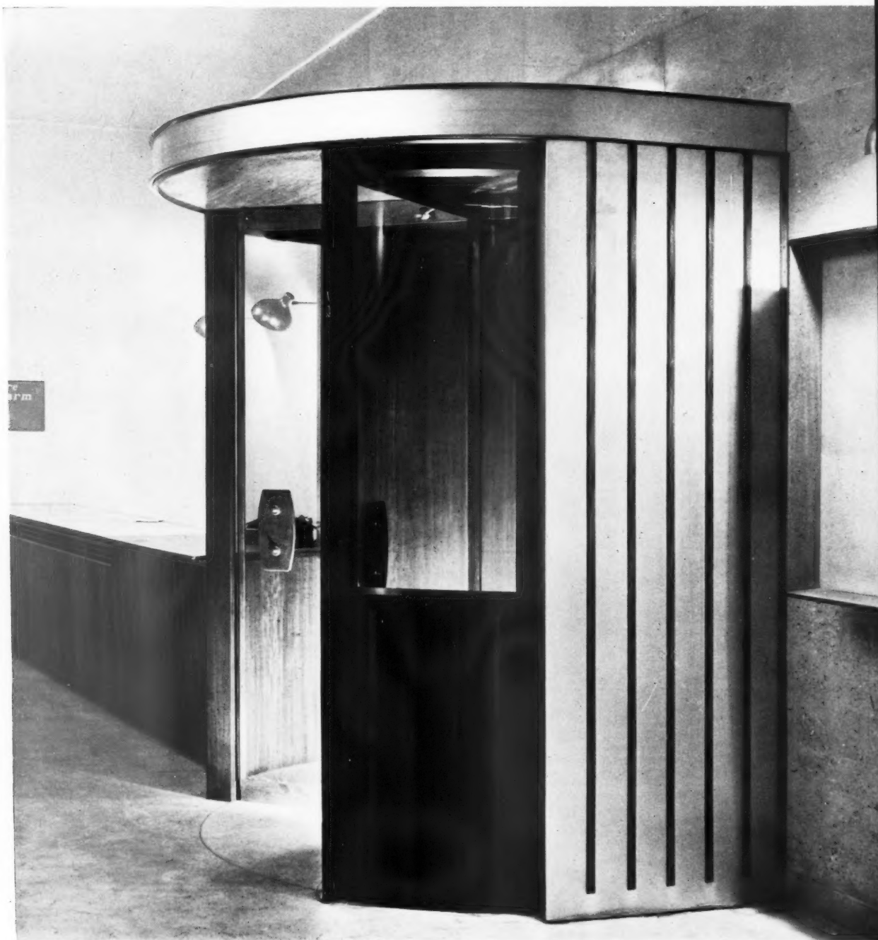
The revolving doors are of armour-plate glass; when not in use they may be folded flat and moved on an overhead track to one side of the opening.
