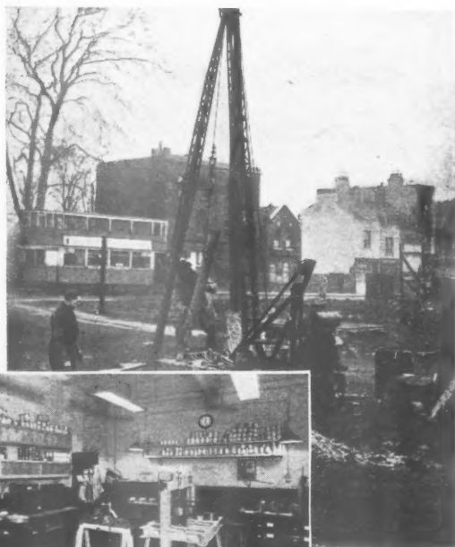
Test boring operations in progress.
