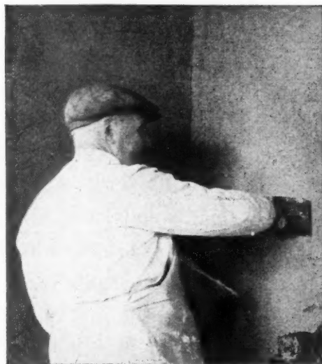
"ZONAPLAX" Undercoat Plaster being applied over brickwork in the usual manner.
