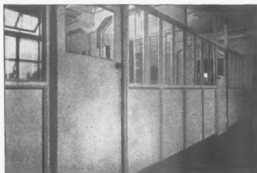
Offices constructed with \frac{3}{8} -in. PLIMBERITE and timber framing, by Messrs. Balger & Co., Confectionery Manufacturers, London, E.1.
