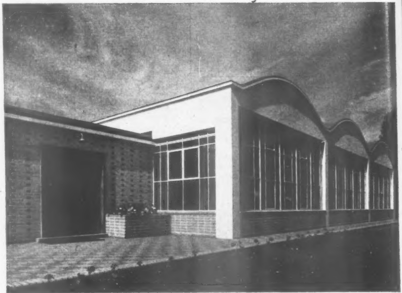
Prestressed concrete barrel vaults for canteen
