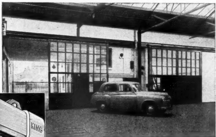
KING Tubular Track, used for the door shown above. It is now made in seven sizes to support doors up to 40 cwt. per leaf.
