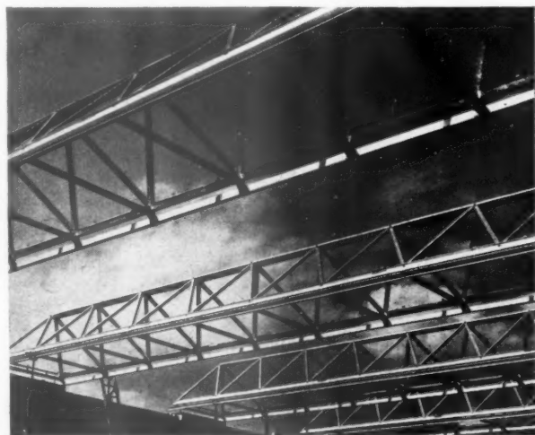
The aluminium space frames used over the stores of the Aero Research factory at Duxford (designed by Ove Arup and Partners).
