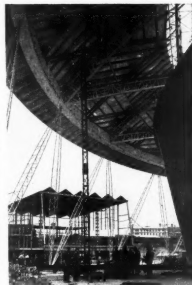
Part of Dome of Discovery during construction, showing the composite nature of the framing—i.e., aluminium alloy roof members and steel ring girder and supports.
