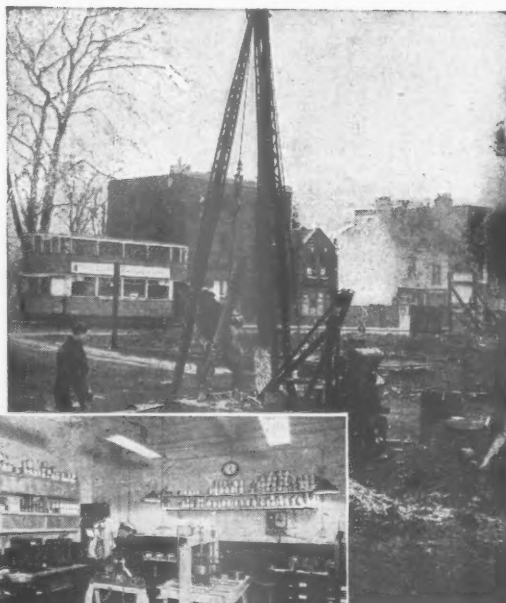
Test boring operations in progress.
