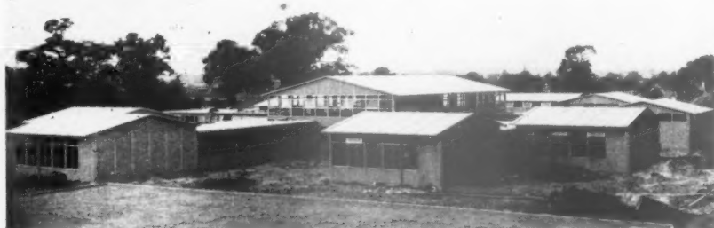
Limbrick Wood County Primary School, Coventry, an example of a system of prefabricated aluminium construction developed by the Bristol Aeroplane Co. in conjunction with the city architect's department, Richard Sheppard & Partners and the MOE. This system is known as the Mark I and is suitable only for single-storey schools. Above, general view of school under construction. Below, interior view showing the incorporation into the system of forms of top lighting and warm-air heating and other items of equipment first developed by the MOE for use at the Wokingham school.
