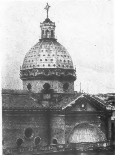
Above, one of the earliest uses of aluminium—the sheet aluminium covering of the semi-cupolas of the church of St. Giocchino, Rome. Below, an important stage in the development of the use of aluminium—a 2-store aluminium prefab.
