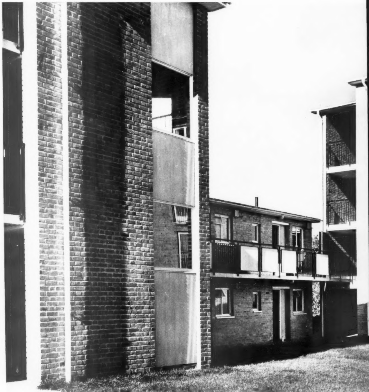
The panel wall, faced externally with fluted asbestos-cement sheeting, is of lightweight construction and has no contact with the edge of the stairs and landings
