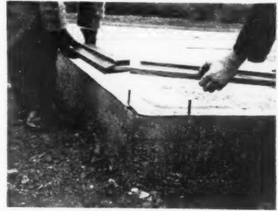
Above, the sill is accurately levelled as the basis of the whole structure. Hardwood strips can be seen, which guide the panels into correct position. Below, posts and panels go up simultaneously. 3 or 4 men can handle the largest sections. Panels serve to brace the frame.
