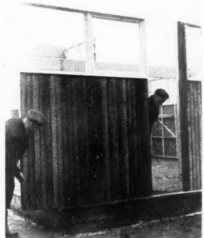
Above, the sill is accurately levelled as the basis of the whole structure. Hardwood strips can be seen, which guide the panels into correct position. Below, posts and panels go up simultaneously. 3 or 4 men can handle the largest sections. Panels serve to brace the frame.
