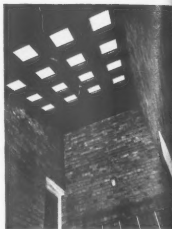
Left, the entrance and staircase block which is constructed of precast concrete blocks finished with a three-dimensional chequer-board pattern. Above, the top of the staircase block. The ceiling is painted deep red. Below, the garden facade and pram store.
