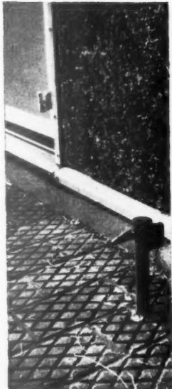
(17) External door holder, made by manufacturers of the doors. It is designed to catch the bottom of the door itself, thereby eliminating the need for cabin hooks, which are difficult to fix and readily damaged, or any similar device.
