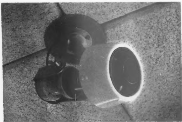
(24) A swivel spotlight, chosen for its adaptability and for its capacity to concentrate light in particular places. When used in conjunction with general lighting, it gives that extra sparkle without which no lighting scheme is complete. The fitting was designed to incorporate a recently marketed 75-watt silvered reflector lamp with a bayonet fixing.
