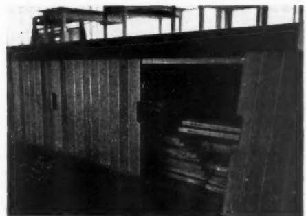
(10) Storage space under the raised side aisles in the hall. One of the panels has been removed and the frames which make up the portable platform units can be seen. These frames which are collapsible, together with their canvas covered tops, are items of standard stage equipment.
