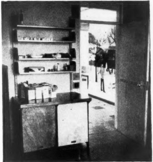
(18) The medical room; ordinary benching and patient shelving has been used. The room is large enough for the prescribed dimension required for eye testing to be obtained. The floor is of chipboard. The door is a standard type of flush door, veneered in hardwood and treated with plastic polish. The door furniture is of anodised aluminium.
