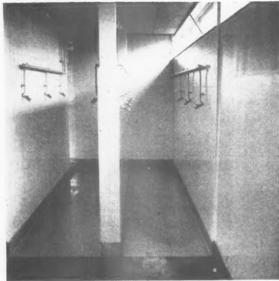
(12) "Run-through" showers of the type used for both boys and girls. One of the few places in the school where glazed wall tiles are used. The floor is of non-slip yellow stud tiles. A single thermostatically-controlled mixing valve regulates the temperature of the water from the sprays. No separate footbaths are provided.
