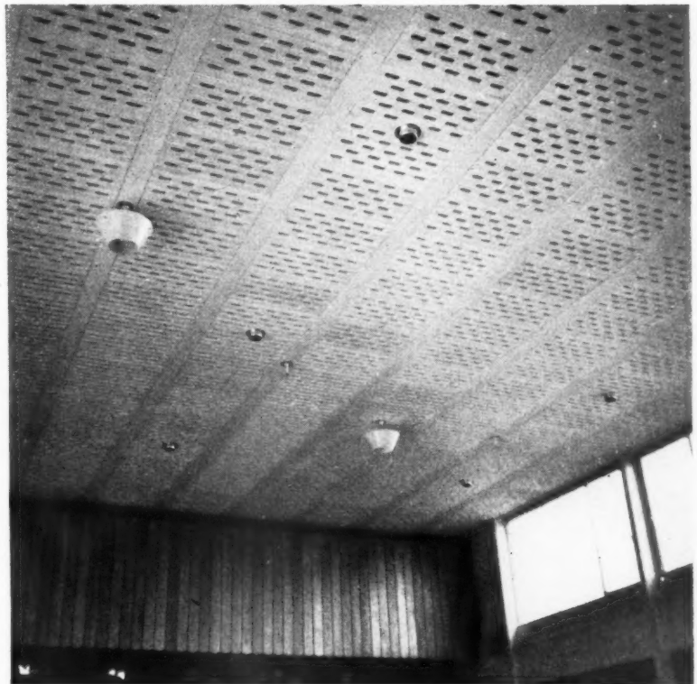
(8) Detail of hall ceiling showing two kinds of light fittings and points for stage spot lanterns. The lanterns are not provided, but are wired for. The fittings with shades are designed to give general illumination—including the ceiling; the others give sparkle.
