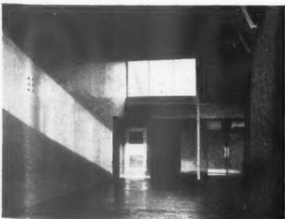
(9) The stage. The rear wall is of plaster panels painted putty colour (Munsell 5·0Y. 8/2). The projecting studs conceal parts of the steel framework. The floor is of Seraya strip. At the far end a typical heater cabinet can be seen. The stage acts also as the circulation area to the gym and changing rooms.
