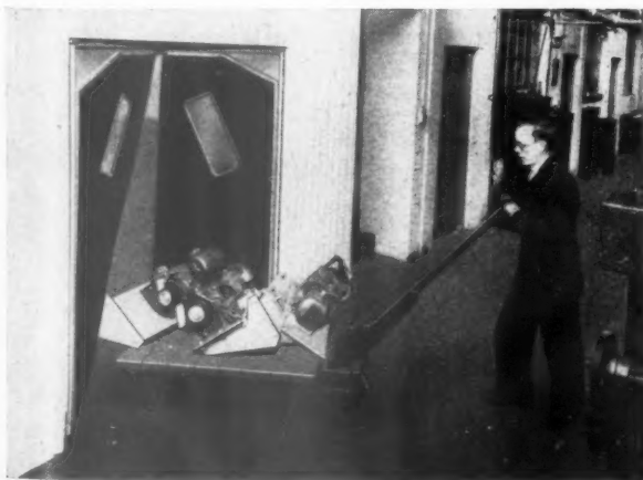
Two uses for rubber in building. Above, D.S.P. carpet mountings for machinery foundations. The section and details show the method of isolating delicate equipment from surrounding forces. Left, flexible rubber doors that may be pushed open by trolleys, etc., without danger or damage.
