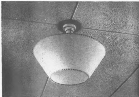
(25) A "Crinothene" shade used in the staff rooms, of similar design to the "Perspex" shade shown in photograph 23. Like the "Perspex" shade, it screens the lamp from direct vision, has an unobstructed downward throw, and allows some light to reach the ceiling.
