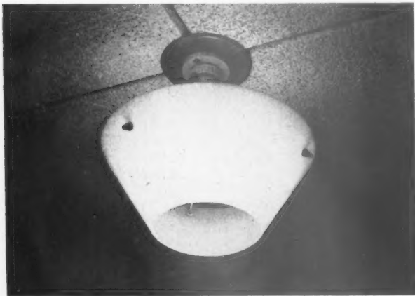
(23) Specially designed light fitting most commonly used in the school. It is simple in design and economical, but fulfils the requirements of shading the bulb from direct vision, and allows some of the light on to the ceiling, in addition to having an unobstructed downward throw. The shade is of "Perspex" specially treated to eliminate glare.
