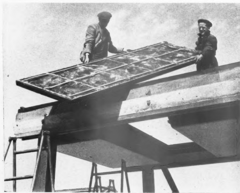
The "Punt" system of construction. Above, details of junctions between the load-bearing wall panels of the Mark II system. Below, the Mark I system; 2 men about to place a ceiling panel between 2 "punts." On the beam in the foreground can be seen the ledge on which the "punts" are supported.
