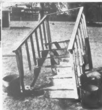
(Alongside) Right half of stairs treated with Albi-"R". Left half untreated. Fires are started simultaneously in two cans of spirit.
