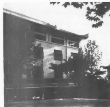
Above, Fig. 4 and, below, Fig. 5, "the placing of traditional roofs on masonry walls"; dormitory block at Wuchang University. Here the architect has attempted to separate the roof from the masonry by introducing large areas of glazing in the top storey.
