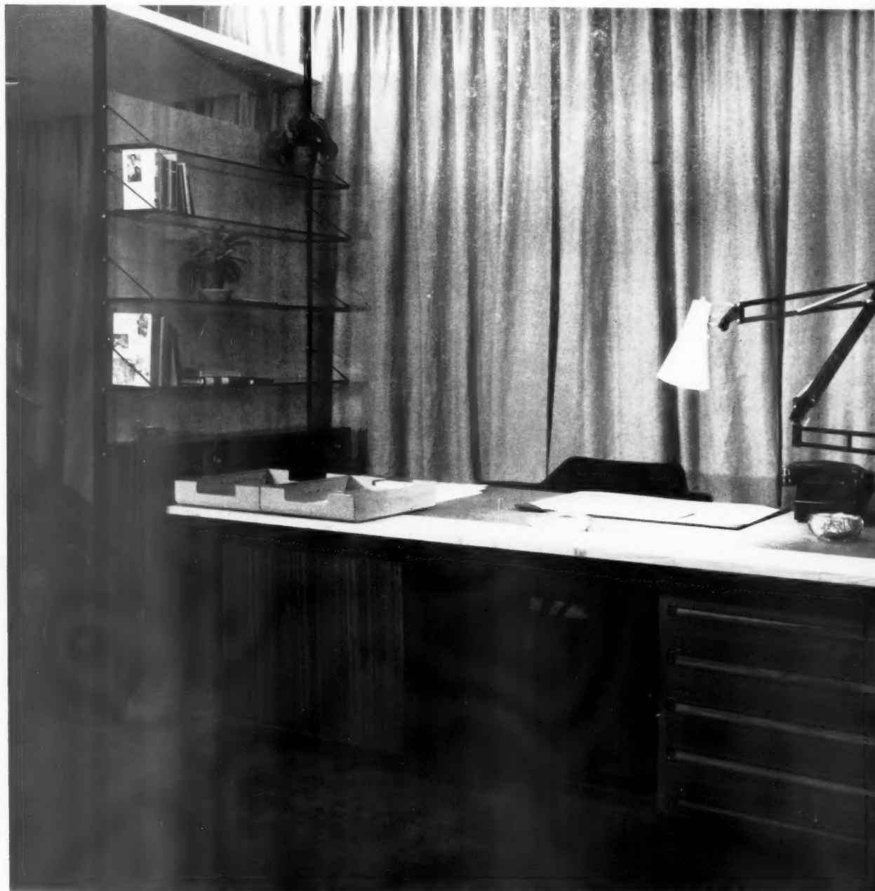
The glass shelves are held by slender brackets to the steel angles which extend from floor to ceiling, supporting the fitting
