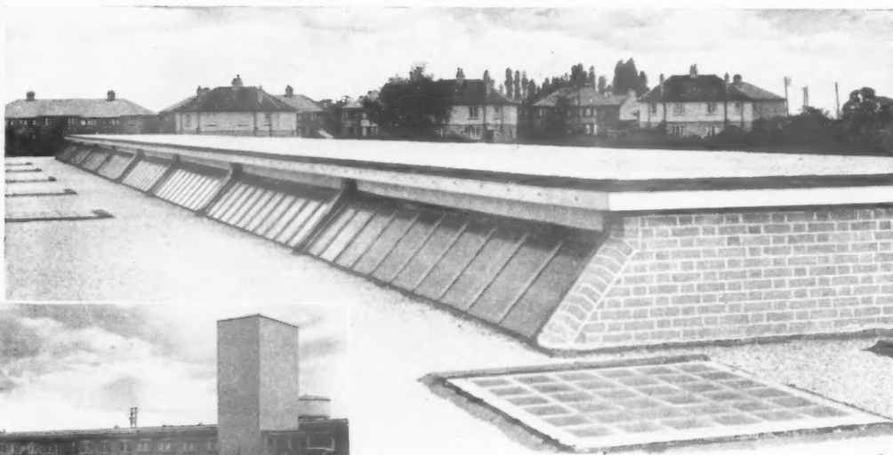
Hatfield Junior School. View of roof screeded with vermiculite.
