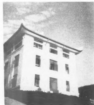
Above, Fig. 4 and, below, Fig. 5, "the placing of traditional roofs on masonry walls"; dormitory block at Wuchang University. Here the architect has attempted to separate the roof from the masonry by introducing large areas of glazing in the top storey.
