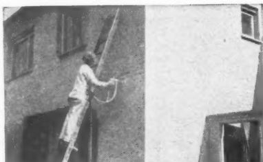
Sealantex Liquid Stone Compound being applied by spray to external walls of housing at Newton Aycliffe New Town.
