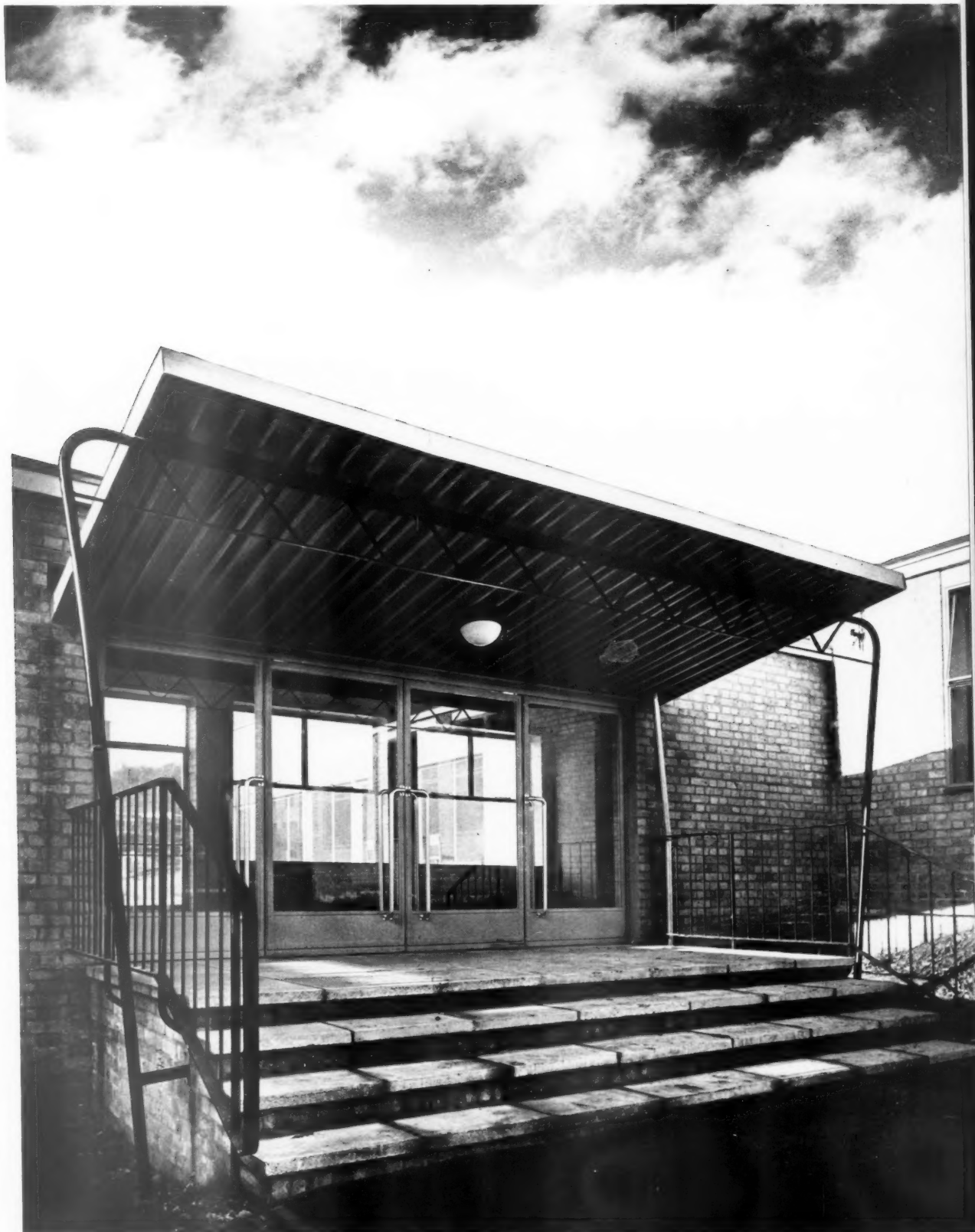
The canopy is of aluminium decking and is supported at the front by a tubular steel frame and at the wall on a steel angle
