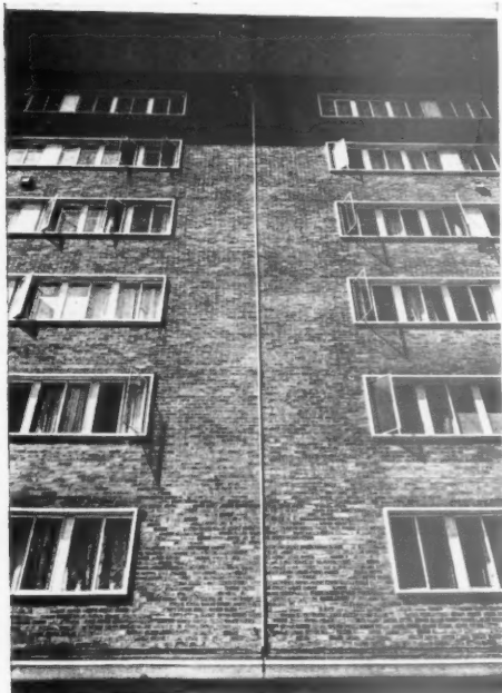
Left, the east facade with expansion joint, which passes through the entire building. Below, the main block, with old people's flats on the left, seen from the south-west.
