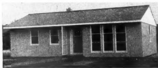
Figs. 19 and 20, Riley-Newsum House (Firm F) as exported to Canada. Designed on a 40-in. module, but not a centre-line module. Most panels, 3 ft 4 in. wide; some, 3 ft 0 1/2 in. wide. Faced with vertical weatherboarding, an additional weatherboard where necessary solves the "thickness" problem.
