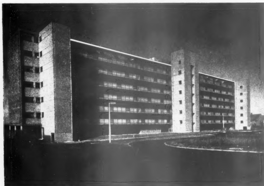
C block from the south-east, showing the access balconies and the staircase (at either end) and lift (in the centre) towers.
