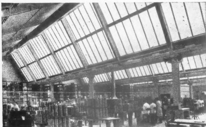
Roof construction showing precast reinforced concrete trusses, purlins and main beams
