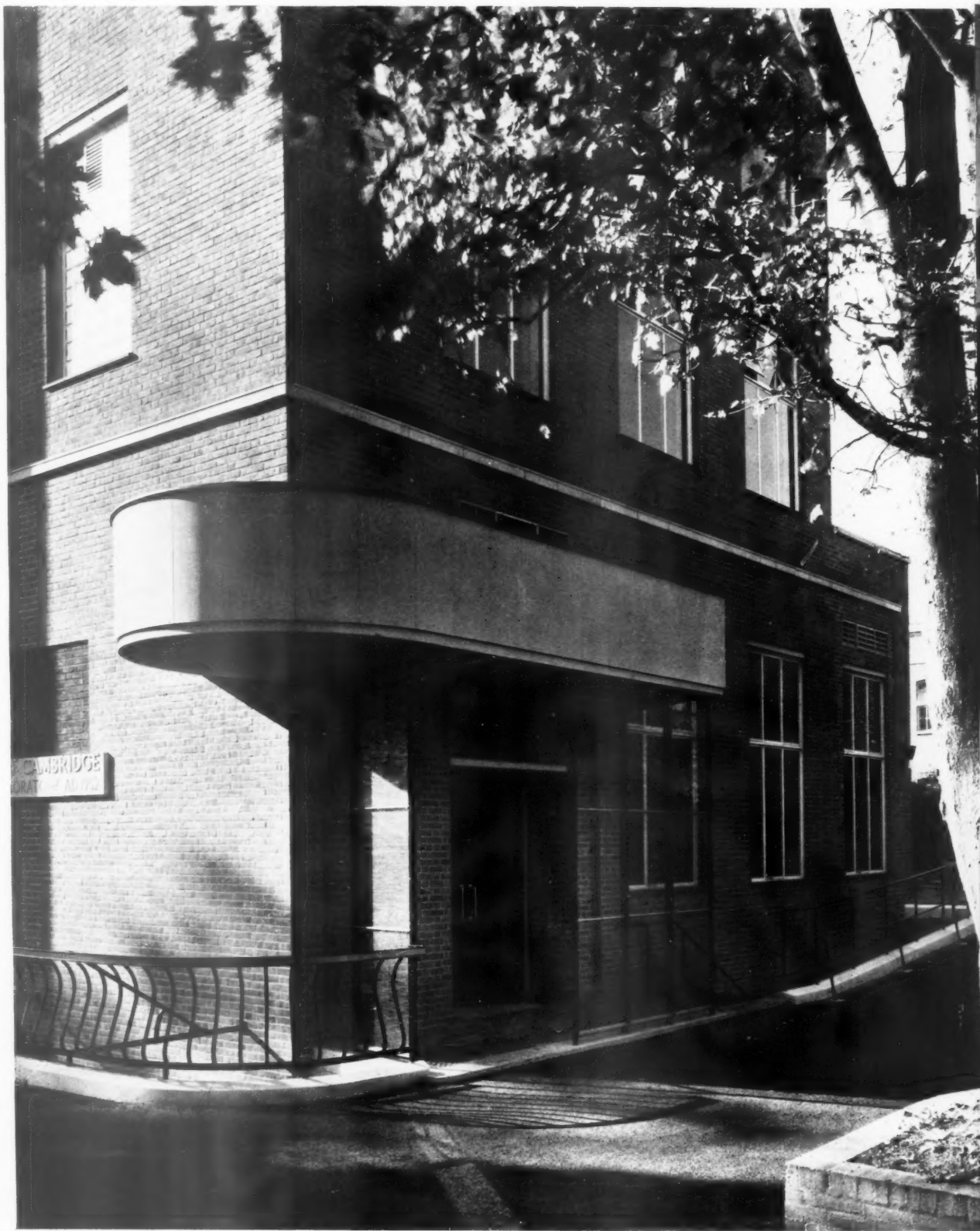
The reinforced concrete balcony is faced with Portland stone and has a lead-lined flower box running round the top
