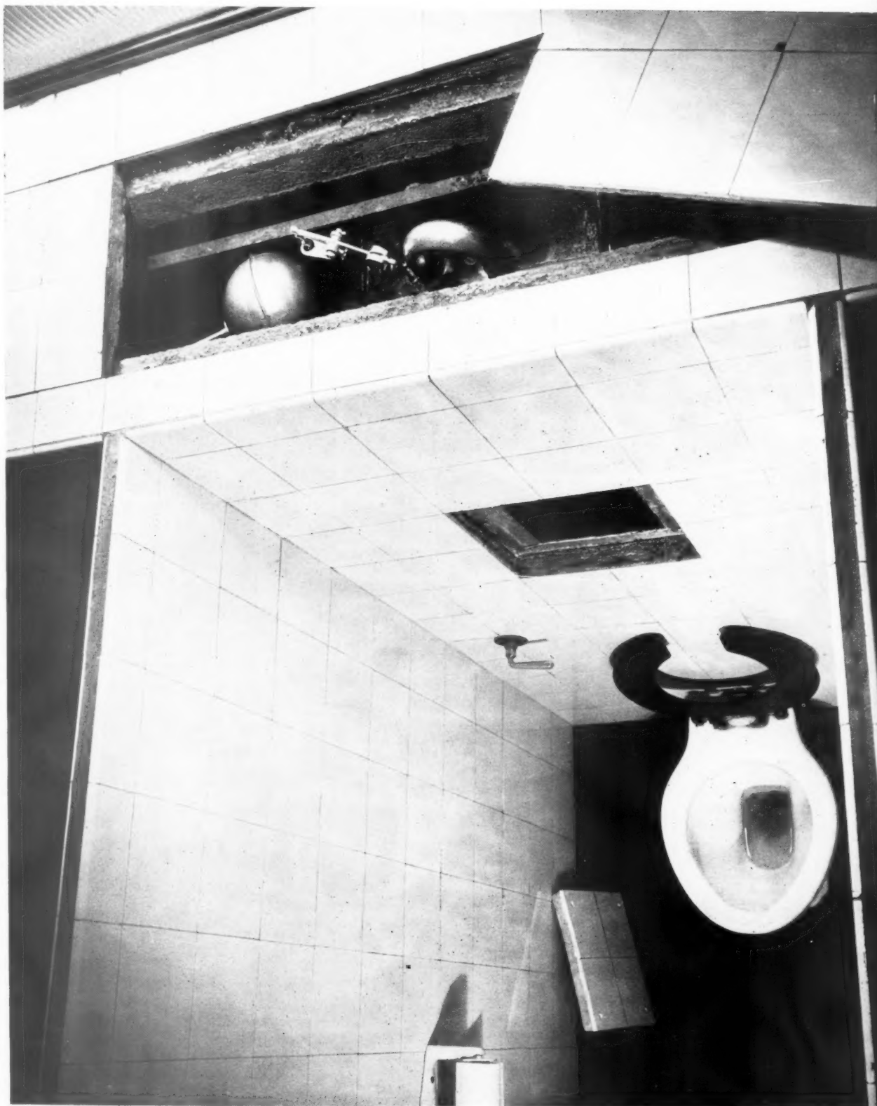
The concealed flushing troughs are accessible by means of removable tile panels
