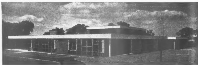
Herts. County Council Summerswood School at Boreham Wood; 40-in. module, with free-standing columns (see photo left, Fig. 11). Below, Fig. 12, general view.
