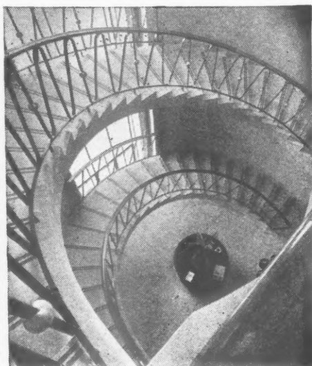
Main staircase of reinforced concrete cantilevered from main frame
