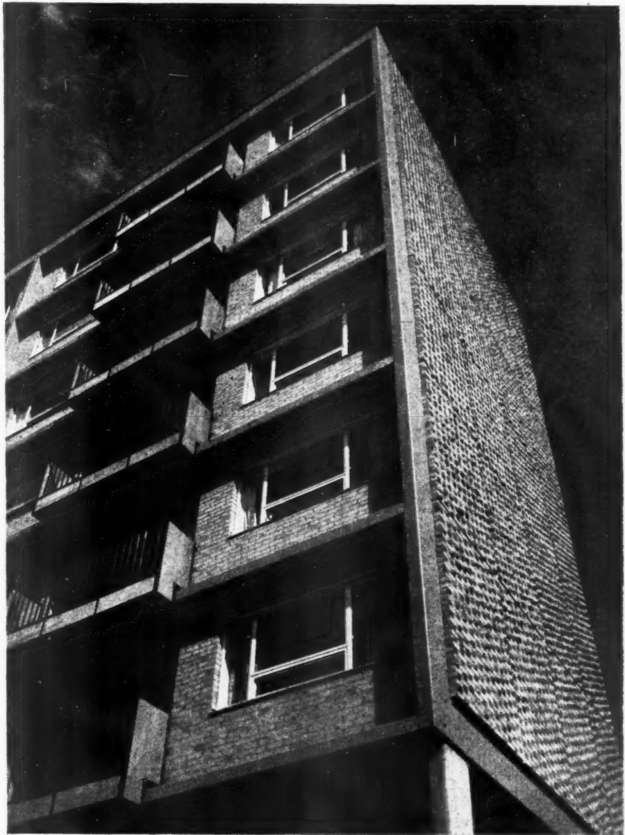
An upward view of the south end of C block. A section on the following page shows how the flank walls are clad outside with panels of 4\frac{1}{2} -in. brick in flemish bond, supported on steel angles bolted to the concrete. The headers are snapped with the snapped ends facing outwards.
