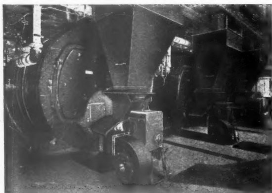
Riley Class 'B' Stokers firing Ruston Horizontal Boilers at a northern hospital.
