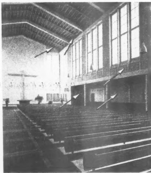
The Markuskirche, Berne (designed by K. Müller and H. Daxelhofer). Extreme left, Fig. 2, looking towards the porch. Left, Fig. 3, looking towards the chancel. The arrows indicate the sound absorber areas.
