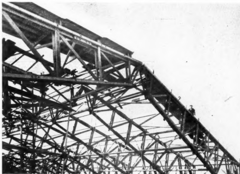
Right, Fig. 8, timber storage shed at Shoreham. Large-span timber trusses, on 3-pin arch system, held together by timber connectors. Below, Fig. 9, close-up of joint at apex of arches.
