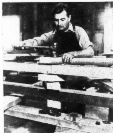
Above, left, Fig. 5, toothed-plate timber connector (double-sided); right, Fig. 6, split-ring timber connector. Right, Fig. 7, building up a truss with timber connectors.
