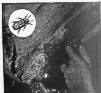
A rofter in the roof of Chichester Cathedral showing damage by the Death Watch Beetle.
