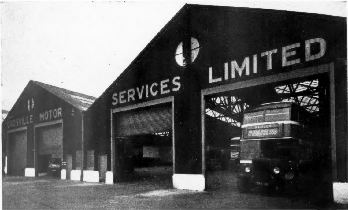
Messrs. Crosville Motor Services, Ltd., Bangor, North Wales Garage, fitted with 4 Kinnear Shutters, each 15' 7" high \times 16' 2" wide.
