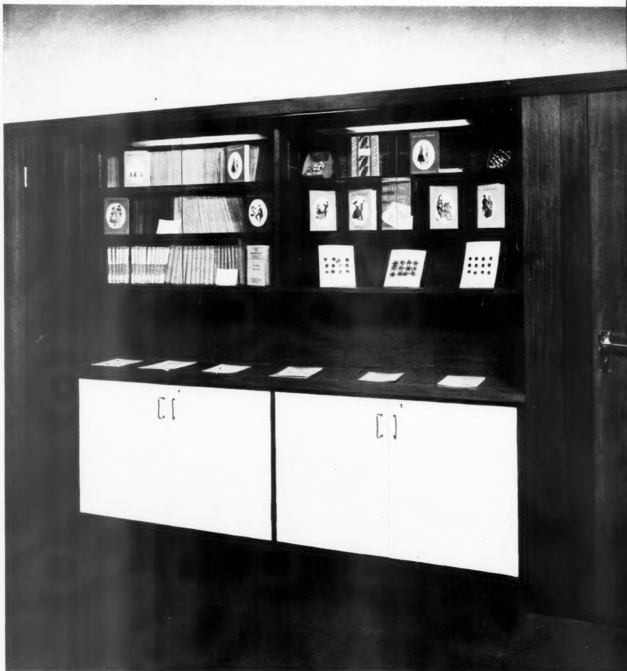
The showcase has glass shelves and sliding doors and is fitted into a recess lined with hardwood: the cupboard doors are of painted blockboard.
