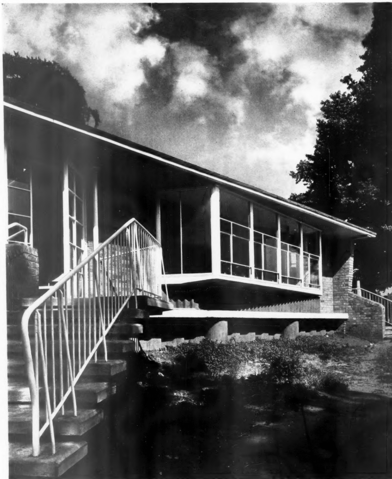
The reinforced concrete cantilever carrying the window forms a wide sill with holes to take flower pots.
