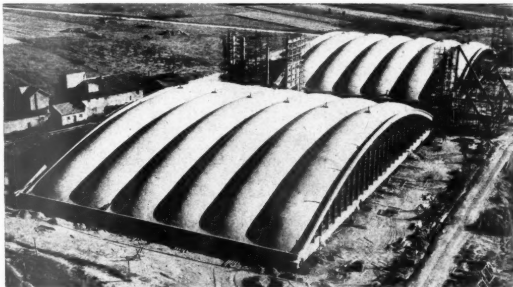
Fig. 4, shell roof at Marignane, France precast on ground and lifted into position (span, 300 ft.). (Photo: Ray Delvert.)
