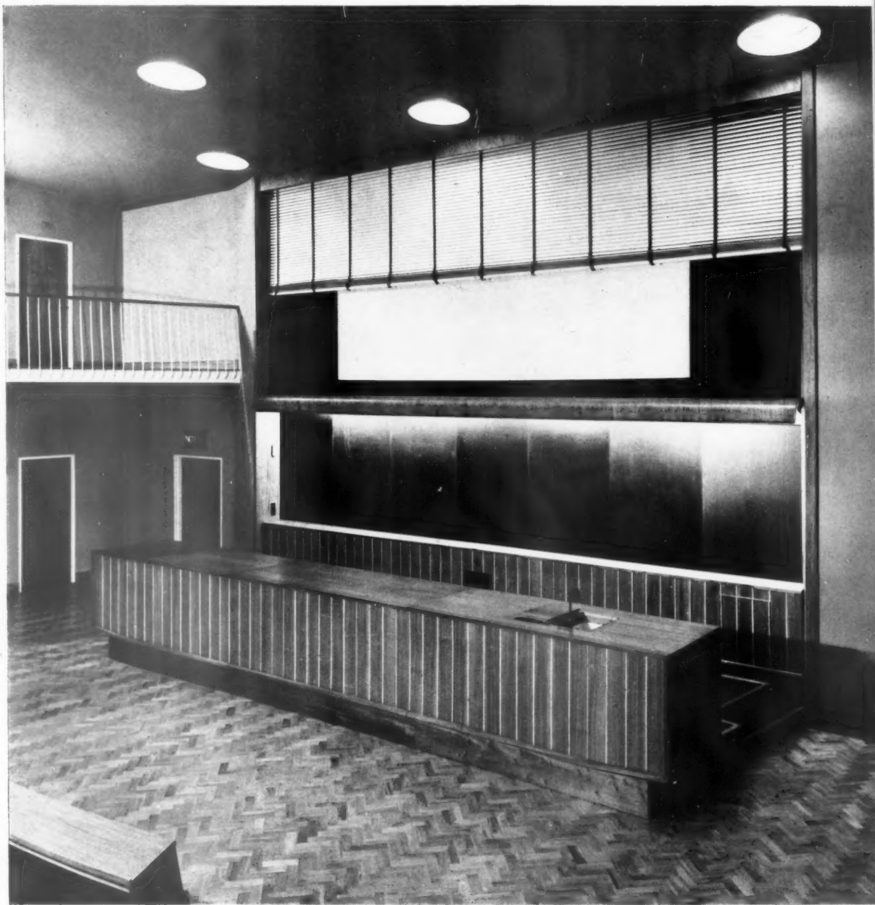
The dais and bench are built in sections so that they may be completely removed.
