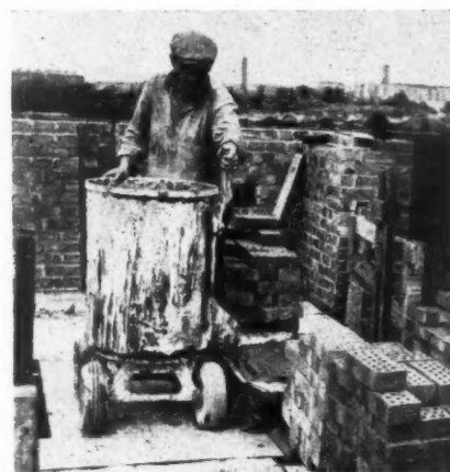
Left, Fig. 5, a popular one-wheel mortar barrow designed to carry 6 buckets, each with a capacity of 0.5 cu. ft. Note the mortar trays: the one on the left is an old wooden model; the one on the right, a new steel one. Note also the steel band round the brick stack; the bricks were delivered from the brickworks ready stacked.
