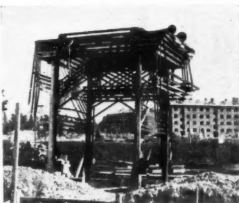
Telescopic platform hoist widely used in Southern Sweden. Above, Fig. 1, the hoist ready to be transported. Right, Fig. 2, the hoist erected. The type shown has two independent narrow platforms; other models have one wide platform.
