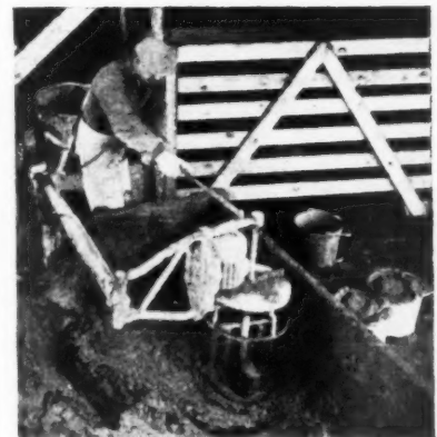
Fig. 7, a device for mixing mortar. Ready-mixed mortar is placed in a box near the hoist. It is stirred up with this machine.
