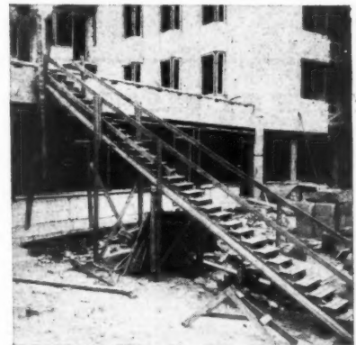
Temporary timber staircases are widely used on Swedish building sites, instead of ladders. Labourers carry large loads of bricks and concrete blocks which could not be carried up ladders. Above, Fig. 10, complete staircase; below, Fig. 11, one section.
