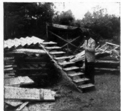
Temporary timber staircases are widely used on Swedish building sites, instead of ladders. Labourers carry large loads of bricks and concrete blocks which could not be carried up ladders. Above, Fig. 10, complete staircase; below, Fig. 11, one section.
