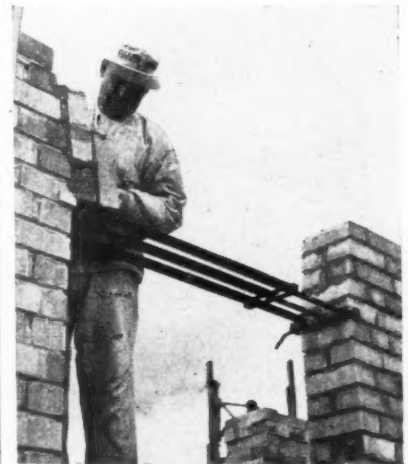
Fig. 6, a new telescopic type of support for flat arches, fastened with wing-nuts at each end. Available in 3 widths, for 1-, 1½- and 2-brick walls.
