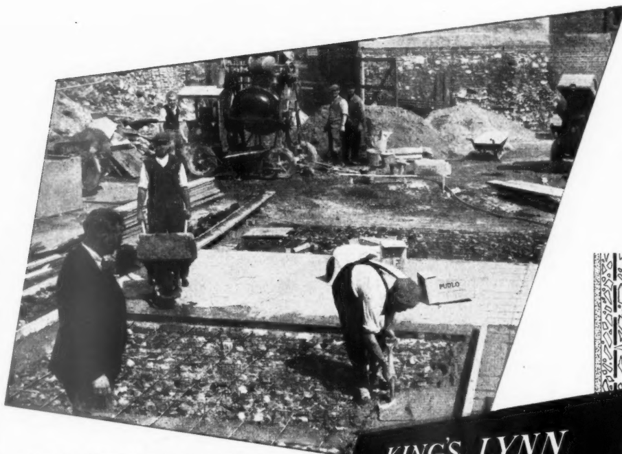
Architect: C. H. Thurston Esq., L.R.I.B.A., F.R.I.C.S. County Architect, 25 Thorpe Road, Norwich. Contractors: Kerridge (Cambridge), Ltd., Sturton Street, Cambridge.
