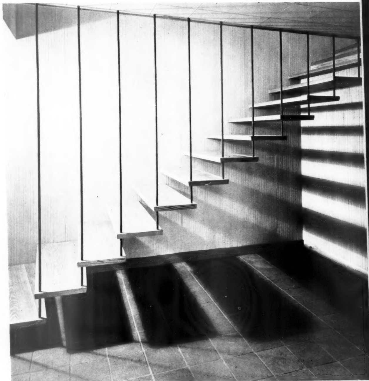
The hardwood treads are supported at the wall on metal angles concealed behind the panelling and at the outer end by the painted rods which completely enclose the staircase.
