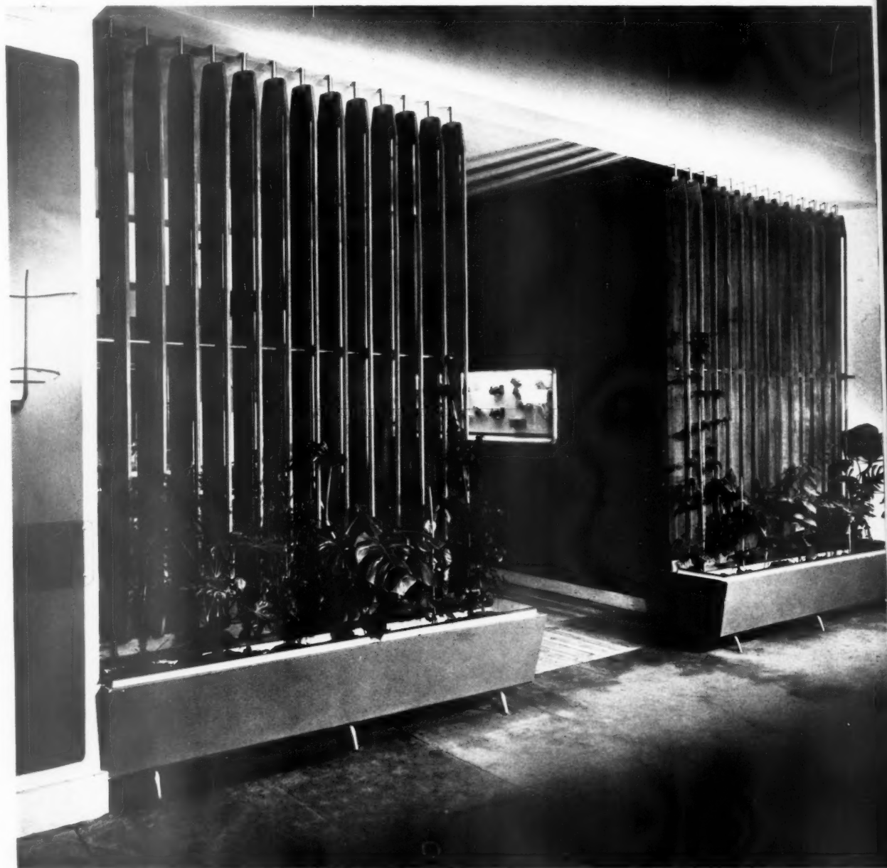
The vertical hardwood louvres of the screen form a support for climbing plants.
