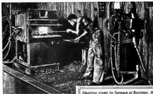
Heating rivets in furnace at Banister, Walton's works, Trafford Park, Manchester.
