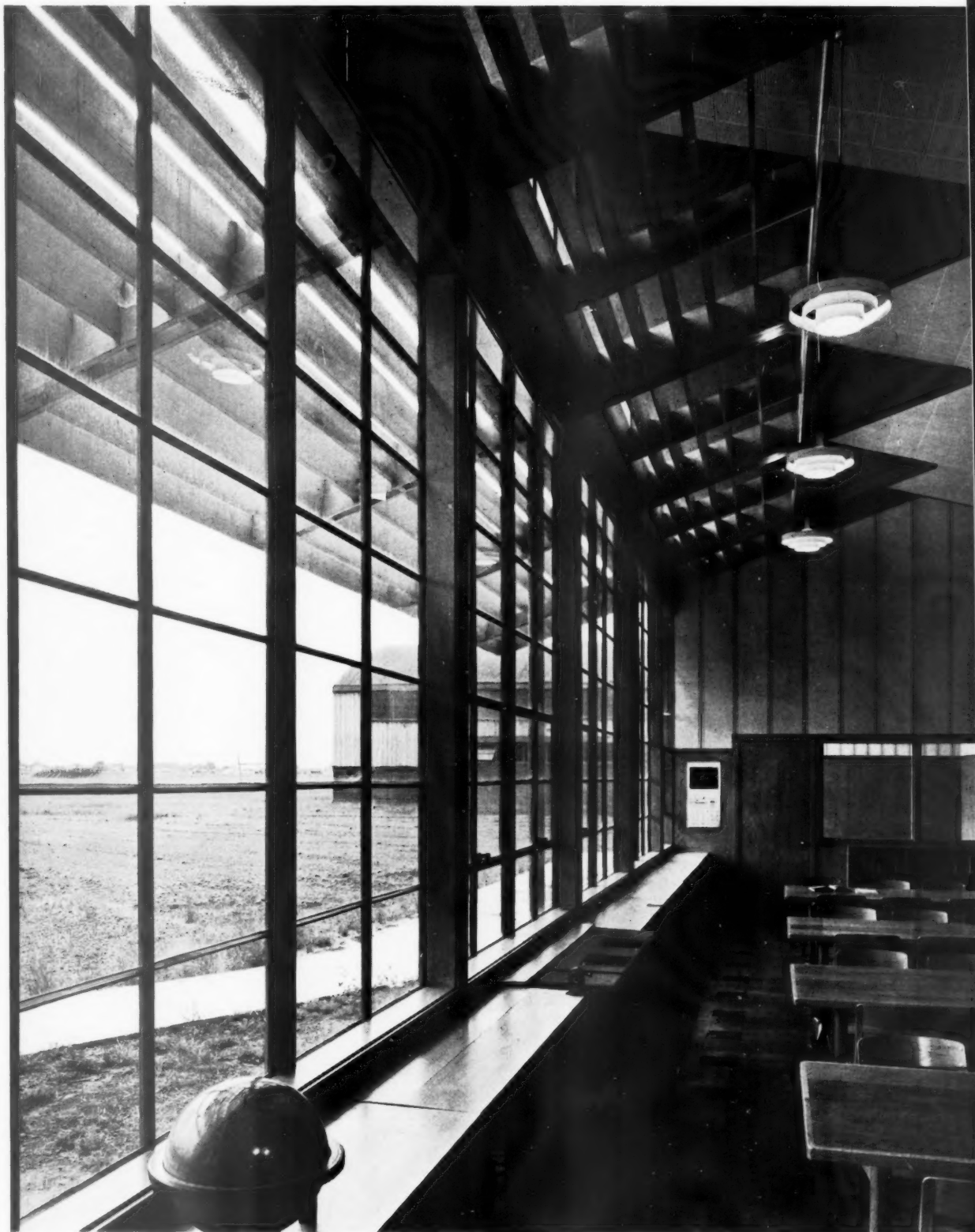
The timber sun baffles controlling the glare from the upper lights are extended outwards to form a screen over the main windows.
