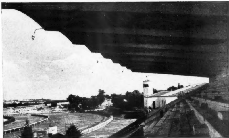
Fig. 7, Madrid Hippodrome stadium, Spain, shells cantilevered 42 ft. from point of support.
