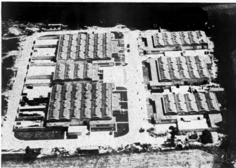
Fig. 1. Aerial view of standard factories at Crawley New Town, all constructed on a 40-ft. by 20-ft. grid, with shell concrete barrel vault roofs.
