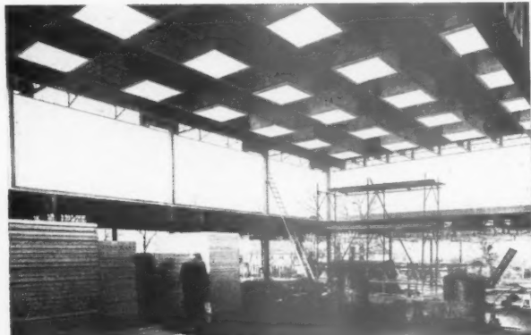
Top, progress on January 21, 1952: the steel frame erected. Above, top lights to assembly hall and wall panels stacked on the site.
