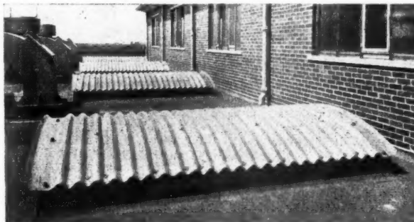
Left, the application of curved corrugated "Perspex" for roof lights. Above, fixing detail for the "Perspex" direct to a kerb.
