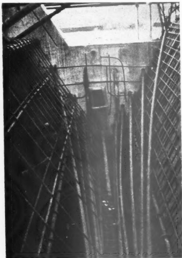
Right, Fig. 7. The position of prestressing cables in a barrel vault without edge beams compared with one with edge beams. Left, Fig. 8. Photograph of prestressing cables in the valley between two shells without an edge beam. Note the high degree of curvature which is possible, as indicated in Fig. 7. Right, Fig. 9. Barrel vault, arched in direction of span, so that prestressing cables can be straight. Below, Fig. 10. Bus garage at Sheffield, covered by thirty 97-ft. 6-in. long prestressed concrete shells, in 3 rows, designed on the principle illustrated in Fig. 9. (Sheffield City Architect's Dept. Consulting engineer, H.G. Cousins.)
