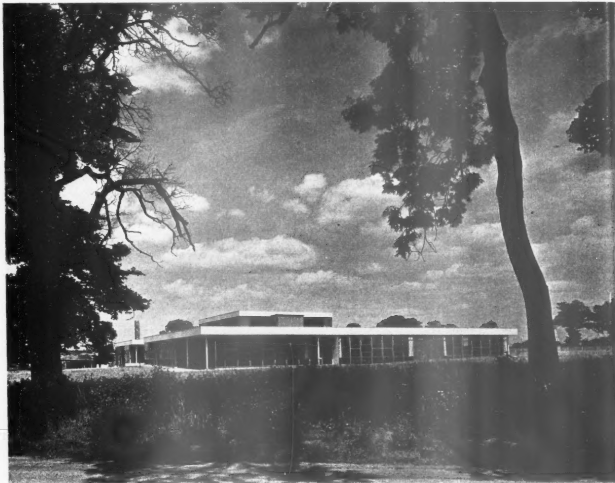
Above, the south and west facades seen from Furze-hill Road.
