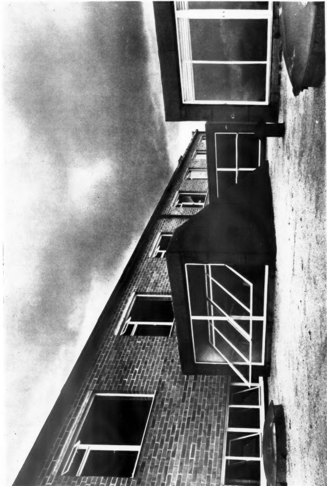
The top and cheeks of the north light structure are cast in one with the roof slab.
