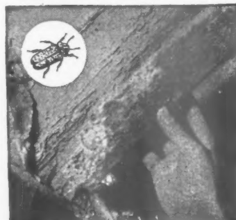
A roofer in the roof of Chichester Cathedral showing damage by the Death Watch Beetle.
