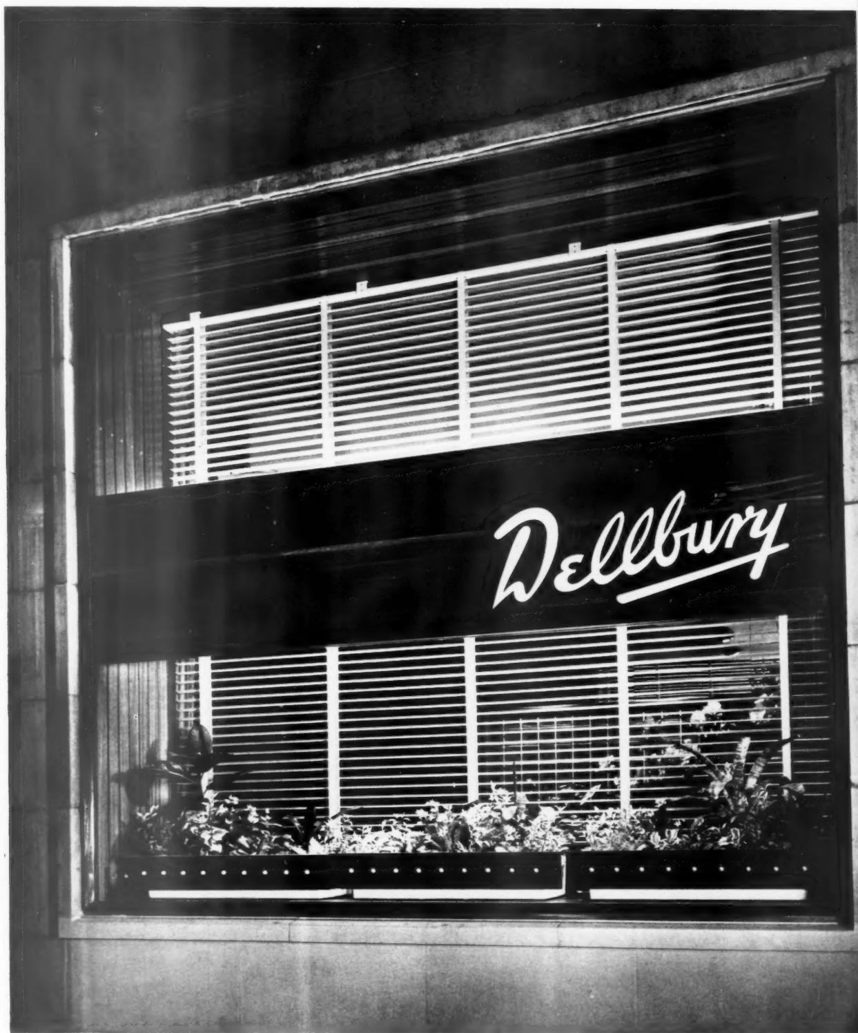
The inside of the window opening is lined with hardwood slats and the glass area is divided horizontally by a panel of similar slats concealing strip lighting.
