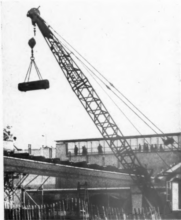
Above, Fig. 1, deflection at centre span; below, Fig. 2, magnified deflection profiles. Left, the bridge being loaded by crane with 3 1/2 ton weights.
