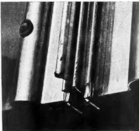
Two close-up views of the fixings of the new aluminium roof at Alexandra Palace (left, from the inside; right, from the outside). Note the die-cast aluminium shoe, specially designed to secure the aluminium glazing bars to the purlins without holes being drilled in the latter. For general view of new roof, see page 67.
