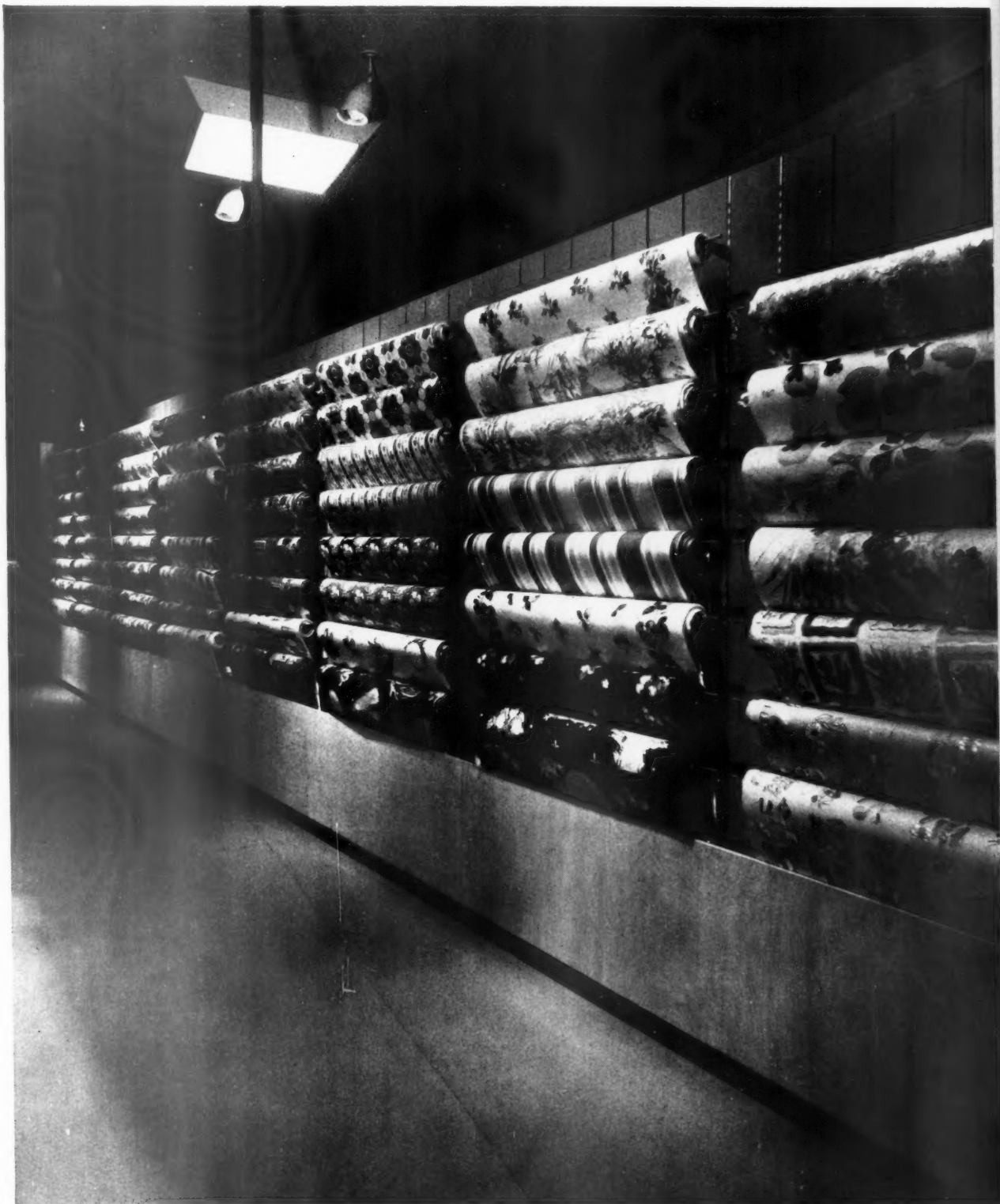
The rods supporting the rolls of fabric rest on brackets which may be adjusted vertically in the slotted metal sections.
