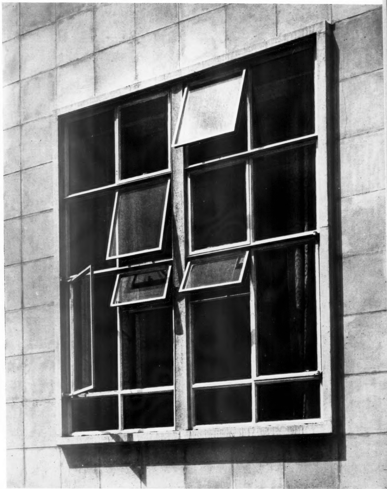
The central mullion of the metal window is made up from two standard transom sections filled with concrete on expanded metal.
