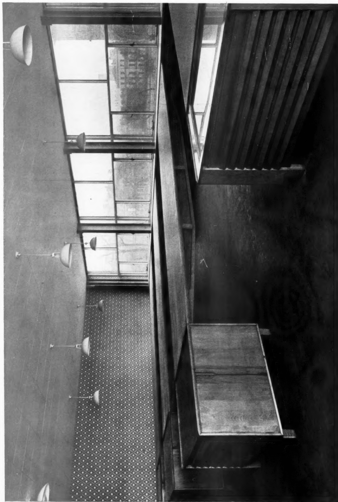
The long drawing tables, supported at their ends only, have been designed to carry a load of 70 lb./sq. ft.
