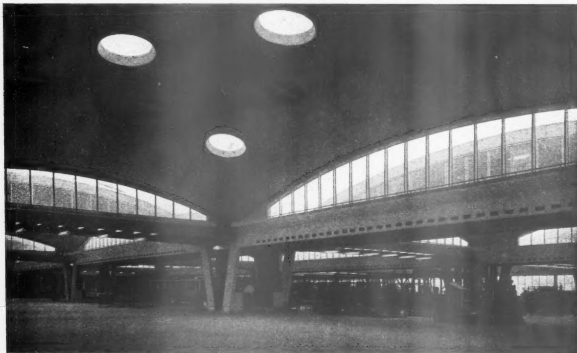
One of the nine shell concrete vaults over the main production area.
