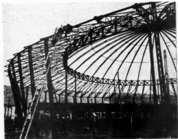
Right, Fig. 5, view of roof construction from below, after dome has been lifted.
