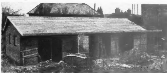
Progress photograph of Robert Townsend's house, showing the construction of the south wall: 2-in. by 2-in. studs and 2-in. wood-wool panels, faced internally with plywood and externally with hardwood boarding.
