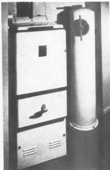
Left, boiler and water softener. Far left, leader controls (bottom), circulation pump (right) and mixer (top right).
