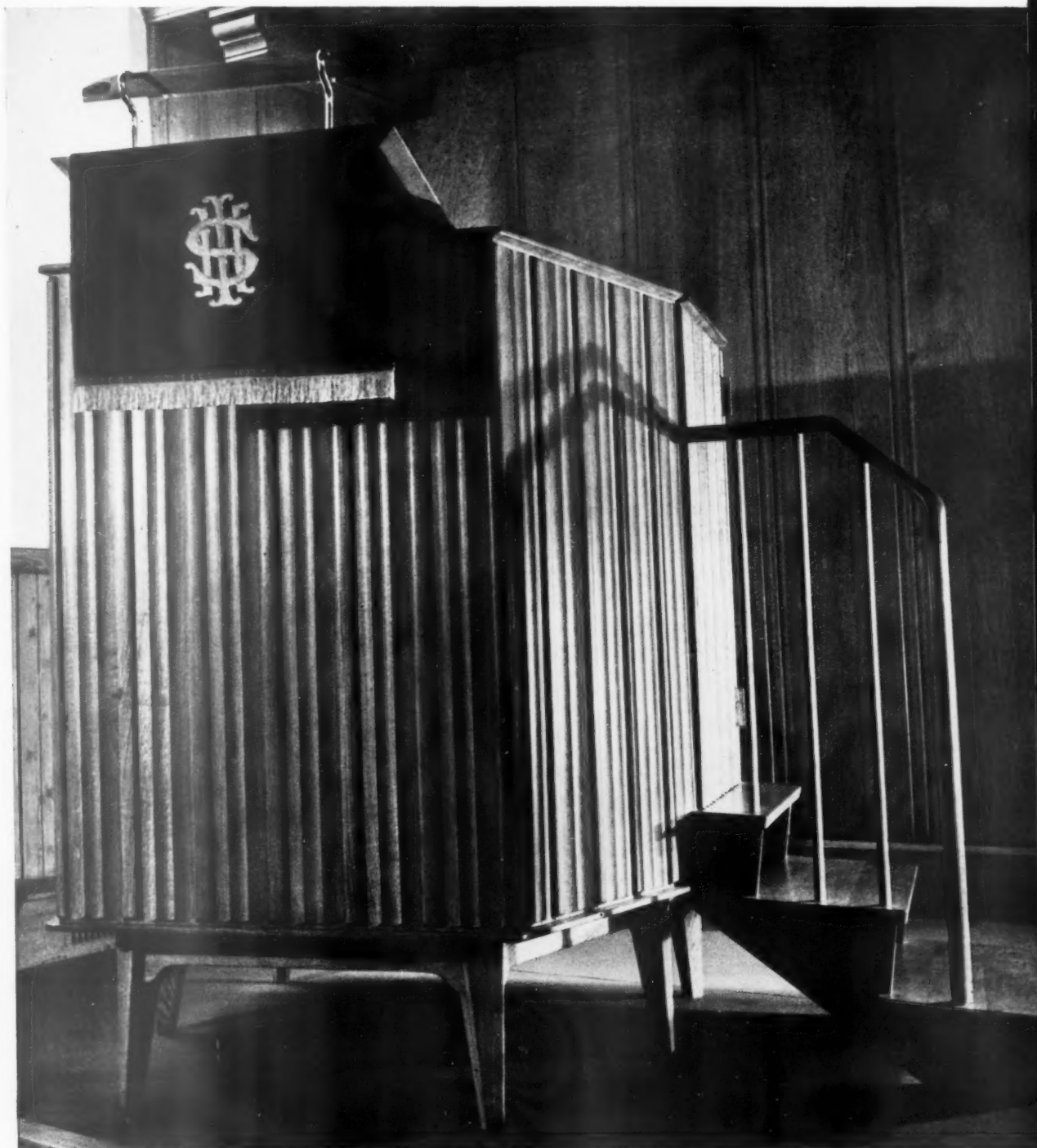
The freestanding pulpit is constructed of oak with moulded panelling and simple balustrade.
