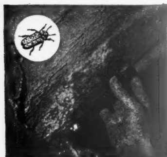
A rofter in the roof of Chichester Cathedral showing damage by the Death Watch Beetle.
