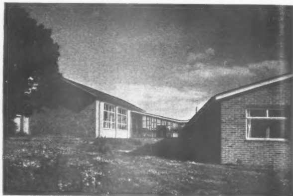
Above, Jean Sheppard's last job finished was a village school, in Little Wymondley, Hertfordshire, for 60 children. Built of traditional materials (exposed hillside position, facing south-west). Construction: walls are of load-bearing brick, relieved by rendering; roof light timber trusses with copper sheeting. There are three classrooms and a hall with a stage, which is also to be used by the village for public occasions. Coloured tiles used to provide permanent colour. The scale is too small for very strong colour, so clear rather subdued tones were used with bright colours for emphasis on some small areas.
