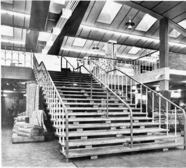
The hardwood treads are carried on three reinforced concrete beams: the balustrade is of tubular steel.
