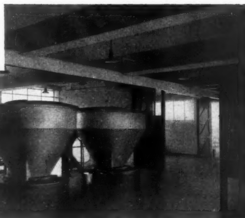
ACID RESISTING POLISHED ASPHALT FLOOR IN FRUIT ESSENCE FACTORY
