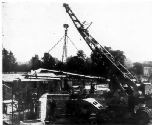
Precast concrete north-light roof trusses (see 19.136). Below, erecting a precast column. Right, hoisting a truss. Bottom right, fixing the purlins.
