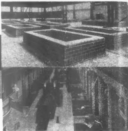
3. Acid resisting flooring in galvanising shop. 4. Prodordur floor tiling in Turbine House.
