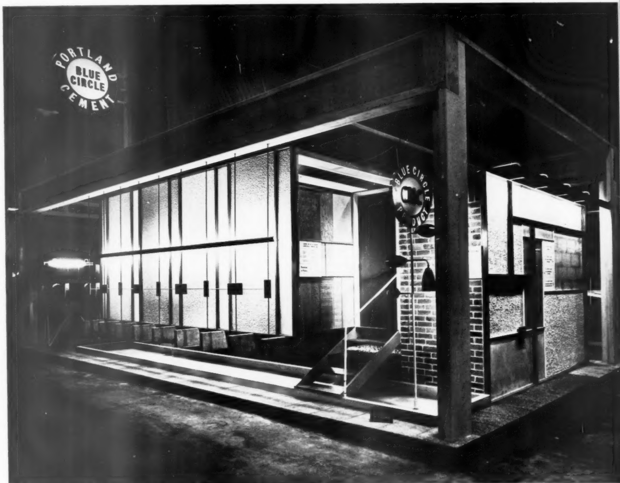
The floor of the stand is suspended by steel wires from a prestressed concrete frame.
