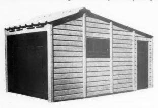
and similar buildings. The standard panels are based on posts at 4-ft. centres and the firm has evolved quite an interesting jig for laying out foundation, a light framework carrying the appropriate core boxes so that when the floor concrete is poured the pier holes are automatically made at the same time. The makers have adopted as a slogan "The charm of the traditional timber building with ten times the life."
