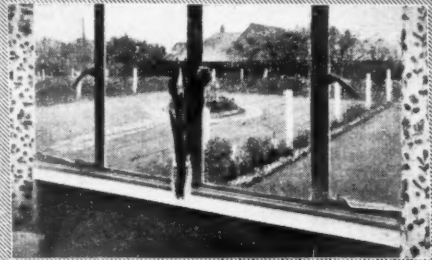
1. A window sill made from a strip of 'Pluto' board.
