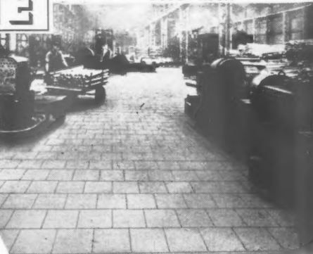
FERROGRAN FLAG FLOOR IN HEAVY EXTRUSION MILL
