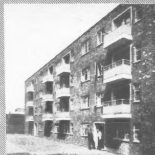
5. \frac{1}{4} in. "Pluto" Board Balcony Panels screwed to mild steel frame.
