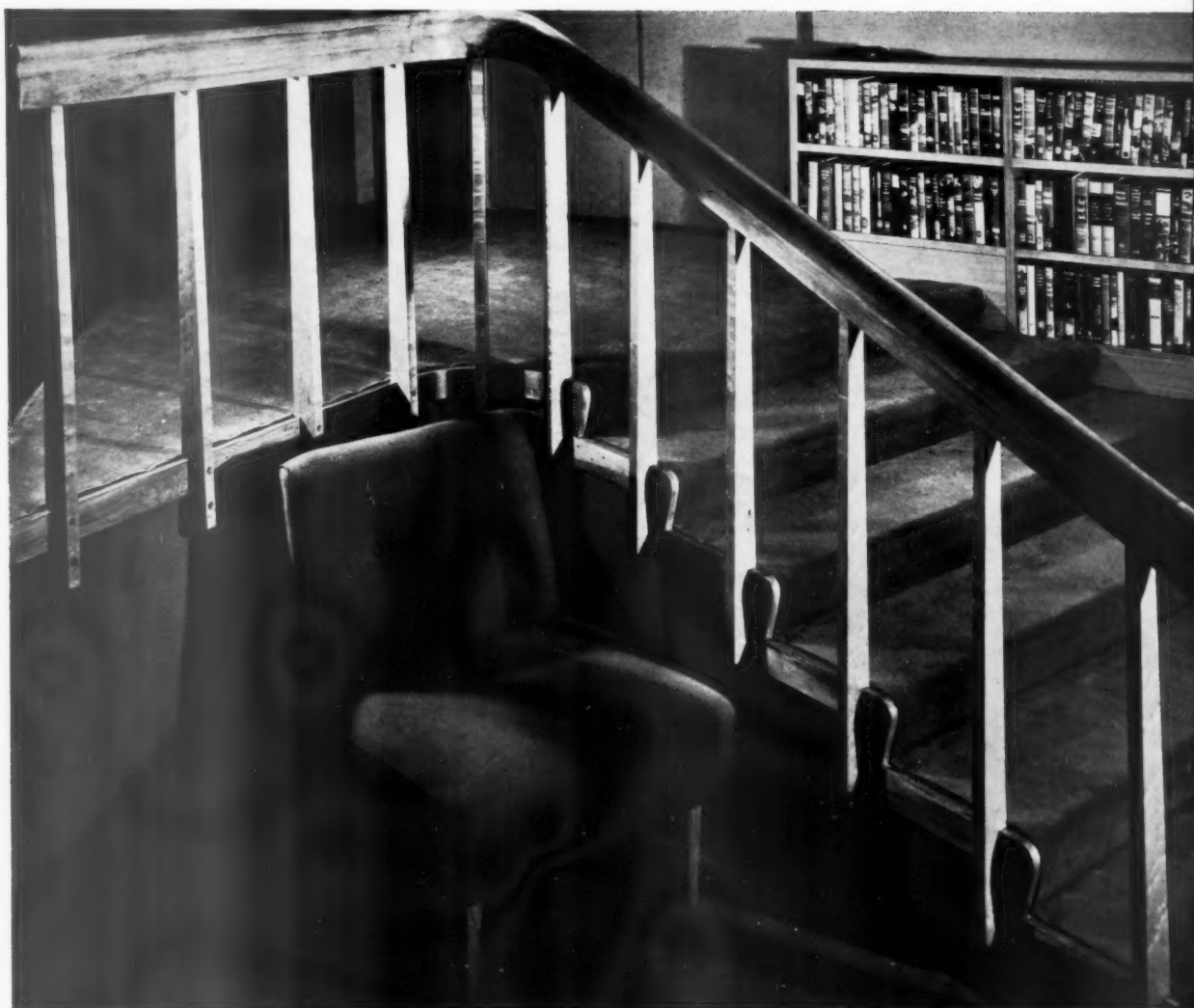
The short flight of shallow steps between two floor levels has a moulded hardwood handrail supported by very simple tapered balusters.
