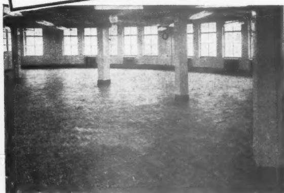
Reconstruction of bomb damaged offices at British Engine, Boiler and Electrical Insurance Co., Ltd. Re-sanded Maple Floor treated with Lignoperm.
