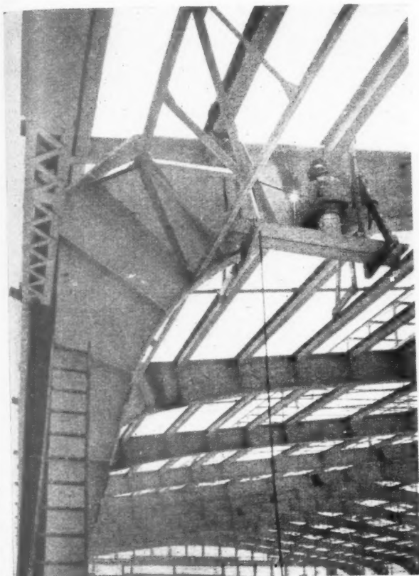
Welder at work on one of the 32 rigid frames supporting the roof of the 200-ft. span harbour shed at Long Beach, California. (See 18.83)
