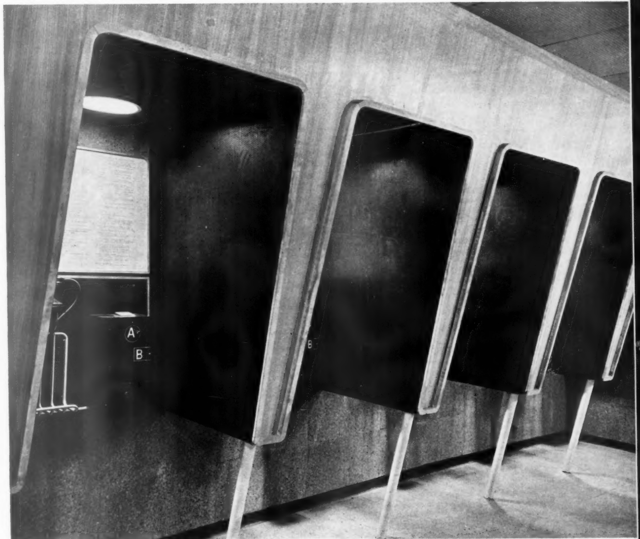
The booths, which are supported on tubular steel columns, are faced on the front with veneered plywood and lined inside with perforated aluminium.
