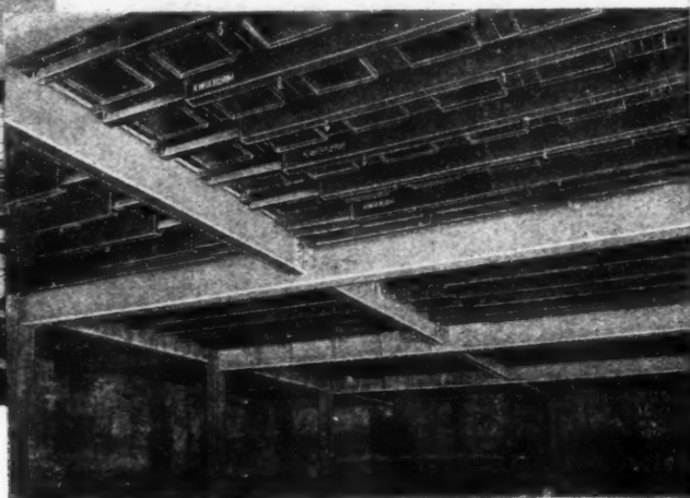
Illustrating the simplicity of laying the Platforms which by their design are held rigidly in position. Striking is equally simple.
