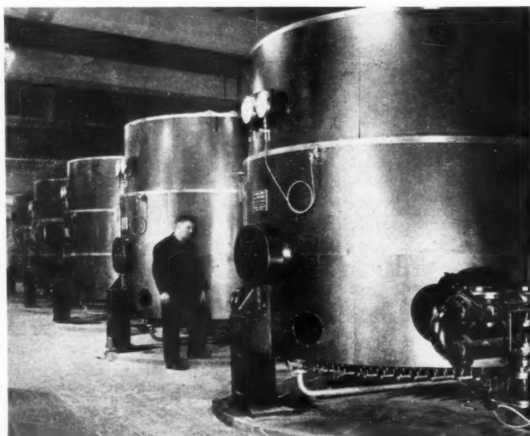
A general view of the boiler house, showing the five gas-fired boilers which serve the heating system.
