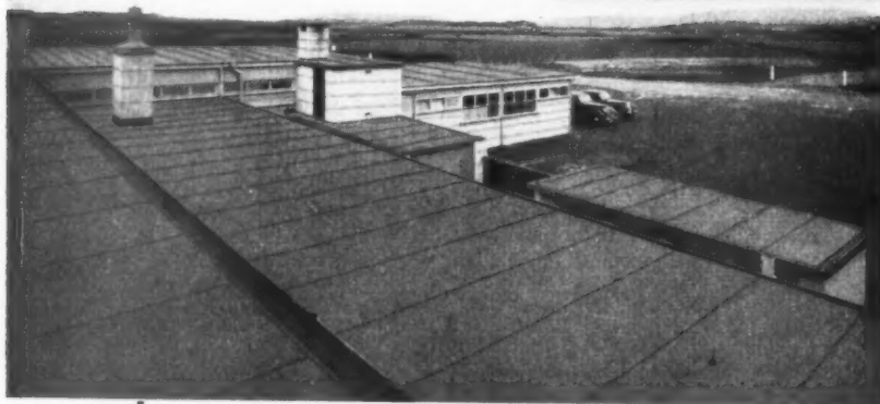
Roof of Ronaldsway Airport, I.O.M. screeded with "KISOL" Vermiculite.
