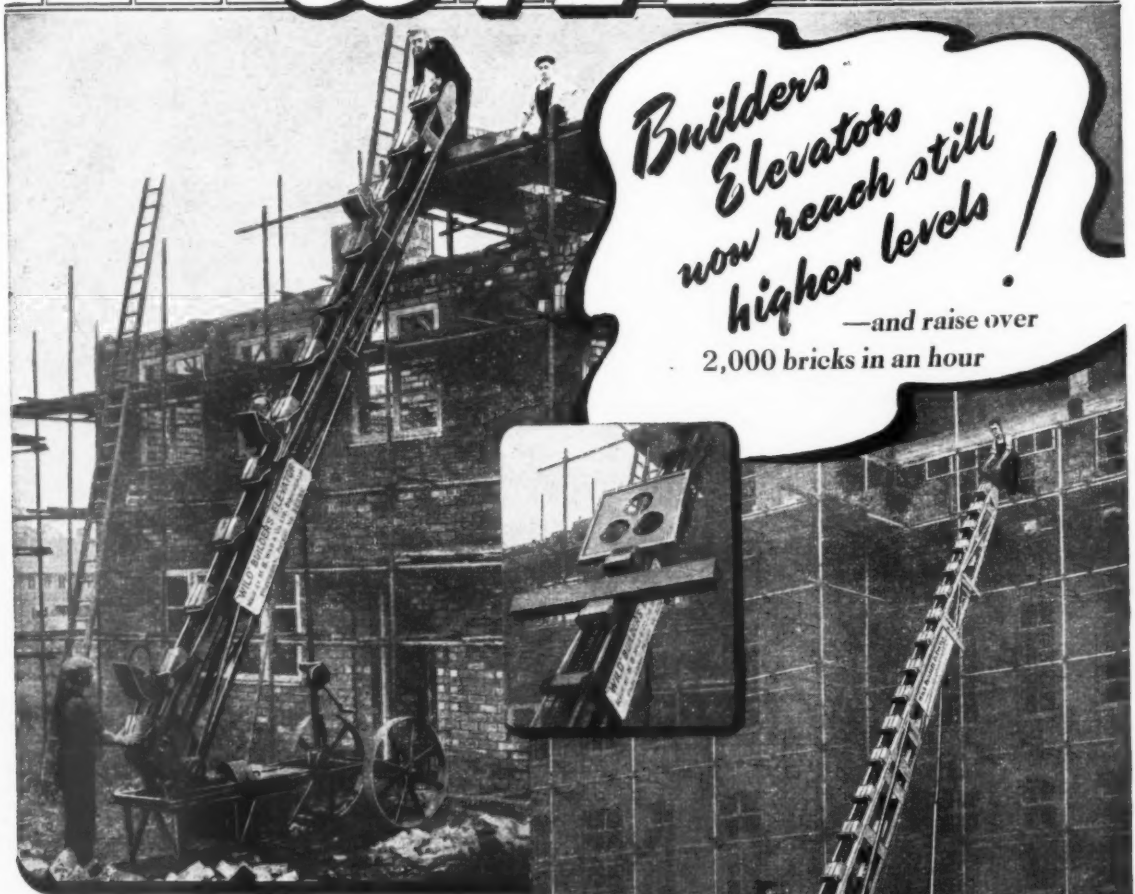
Standard "Wild" Elevator in use at a housing site. Note the mortar buckets.
