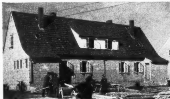
Refugees in Bremen building their own homes, using interlocking cavity blocks (right) made with high percentage of coarse sand and lined with fairly wide horizontal mortar joints. Walls finally plastered inside and out; open joints form good key for plaster.
