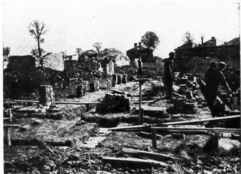
Experimental housing site at Northolt. Dudley rural houses being erected by MOW mobile labour force and observed for time and motion study. Site progress by 16th day (April 12, 1944).
