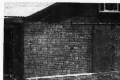
Fig. 9, walling of concrete blocks with crushed stone aggregate.
