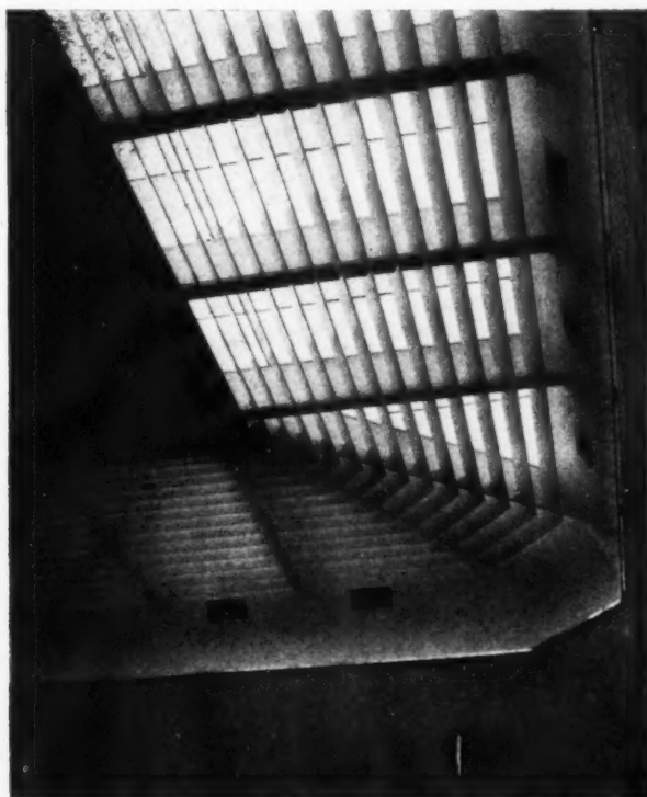
Fig. 11, inclined louvres in the ceilings of the main picture rooms at the Boymans Museum.
