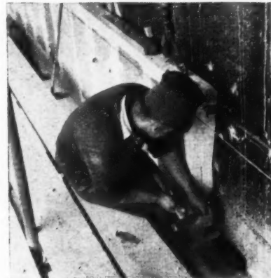
Top left, the lowest course of the Portland stone facing slabs stacked (upside down) before erection. The drip, the rebate and vertical slot are clearly visible. Top right, the RC nib designed to support the external stone slabbing. It also shows horizontal and vertical GI dovetail channels. Above left, fixing cramps and setting slab into position. Above right, a section of stone facing fixed away from the concrete wall with long cramps.
