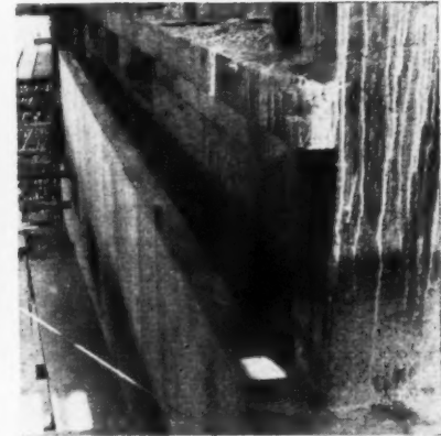
Top left, the lowest course of the Portland stone facing slabs stacked (upside down) before erection. The drip, the rebate and vertical slot are clearly visible. Top right, the RC nib designed to support the external stone slabbing. It also shows horizontal and vertical GI dovetail channels. Above left, fixing cramps and setting slab into position. Above right, a section of stone facing fixed away from the concrete wall with long cramps.
