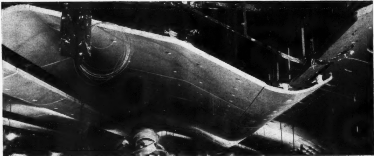
Fibrous plaster ceiling to auditorium nearing completion. The supporting metalwork is largely site welded. (Official photograph.)
