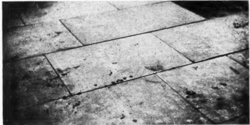
Artificial stone paving to floor of entrance hall at 12 level.
