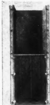
(Left and above left) The use of Milforms for wall shuttering with angle-iron wallings and "Rawlties". This shuttering is self-supporting and automatically aligning. A light access-scaffold only would be required in addition to the above items.
