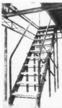
Built at Mills' Birmingham Depot. A prefabricated staircase, light and easy to handle: a stout and rigid structure when erected.
