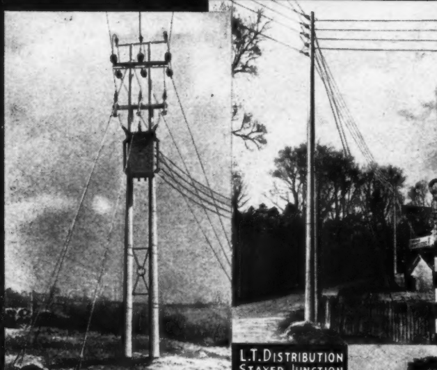
6.6 KV. OVERHEAD LINE TRANSFORMER STRUCTURE
