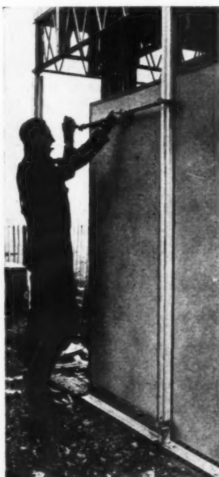
Fixing, left, a plastic panel and right, an aluminium extrusion. The mastic tape caused such a tight fit that a cramp had to be used.
