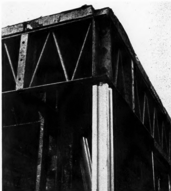
"Close-up" at roof level, showing the perimeter beam cantilevered out from the framing. Note spigot fixing for aluminium extrusion to allow for thermal movement.
