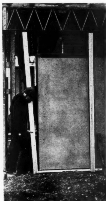
Fixing, left, a plastic panel and right, an aluminium extrusion. The mastic tape caused such a tight fit that a cramp had to be used.
