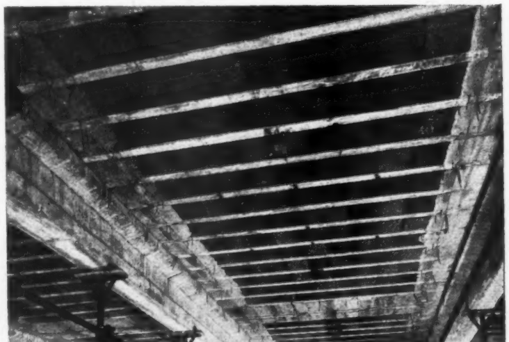
Completed floor, before removal of props.
