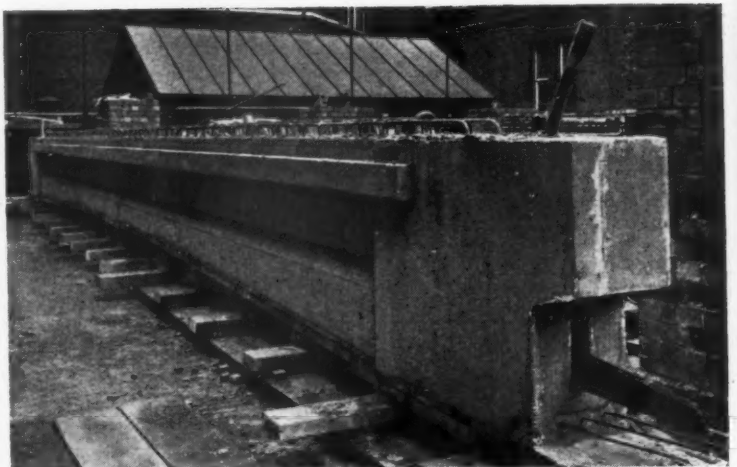
Typical main beam prior to prestressing.
