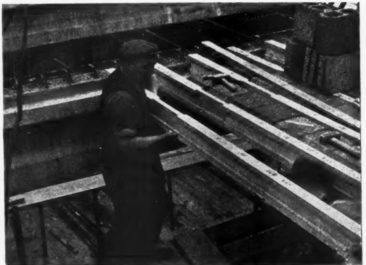
Laying precast ribs and hollow block floor.
